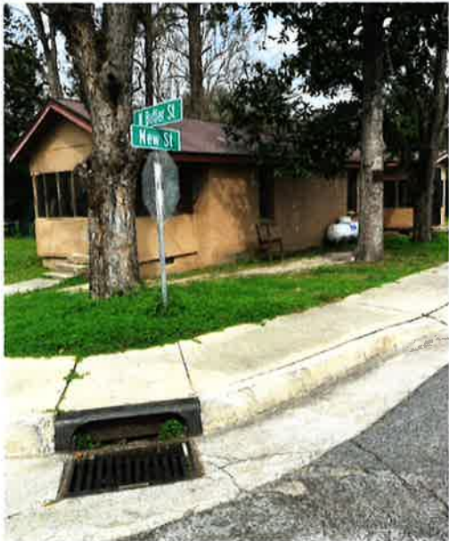
Homes located on North Butler Street
