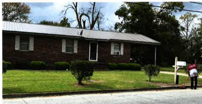
156 North Harney Street
